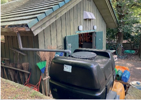
Harvesting rainwater & using this to clean tools at Yokohama War Cemetery (Japan) (left & centre); at Brookwood Military Cemetery (UK) (right), the installed rainwater harvesting system will provide water to support both the plants in our small nursery & the establishment of plants & trees around the site.
