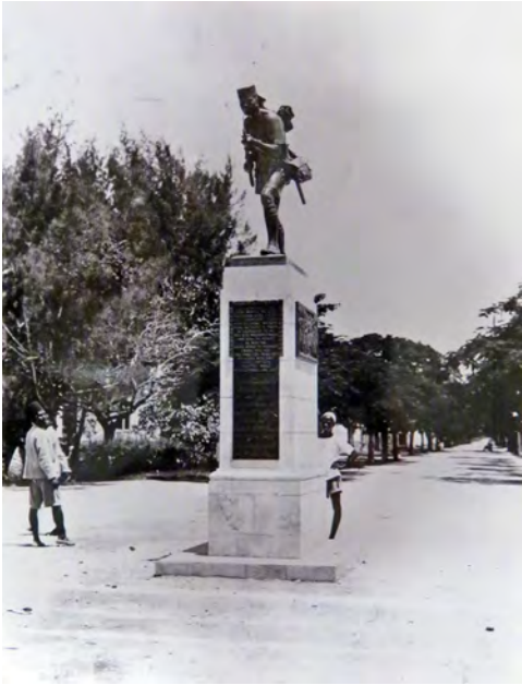
Photograph of the front of the completed memorial in place, 1928
