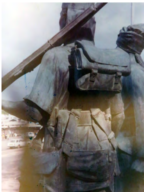
Pre-renovation detail of the back of the King's African Rifleman, 1973
