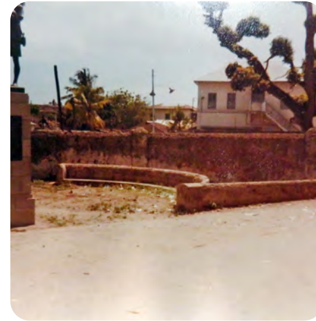
The low wall and seat were chipped and there was no planting, 1979
