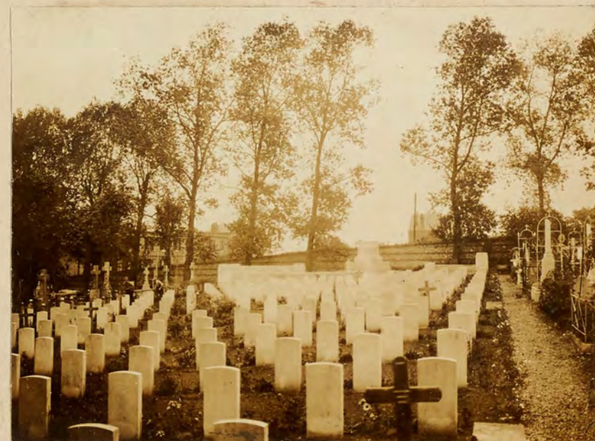
CROSS WAITING ERECTION NEW MONOLITH SHAFT.
