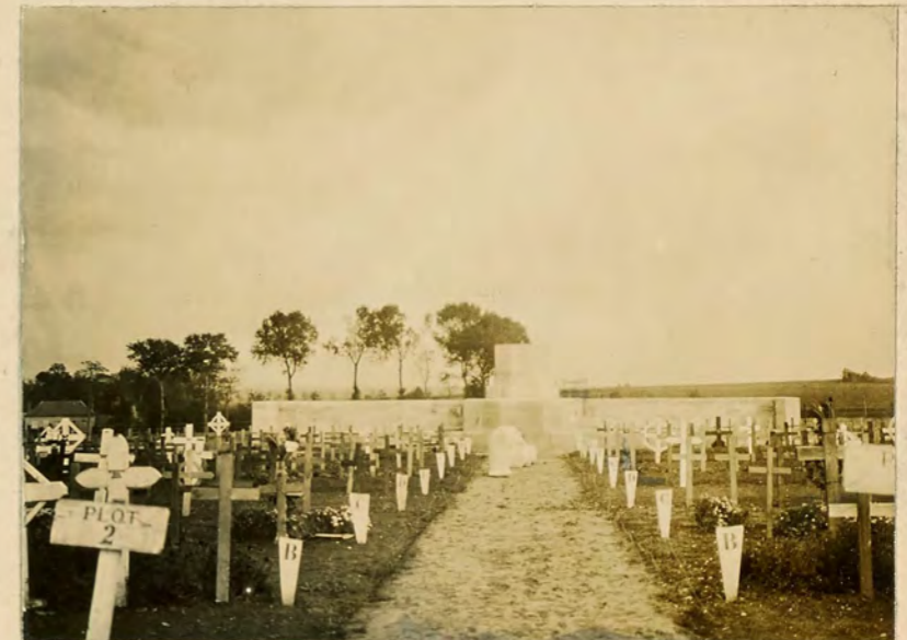
CROSS BEING ERECTED
