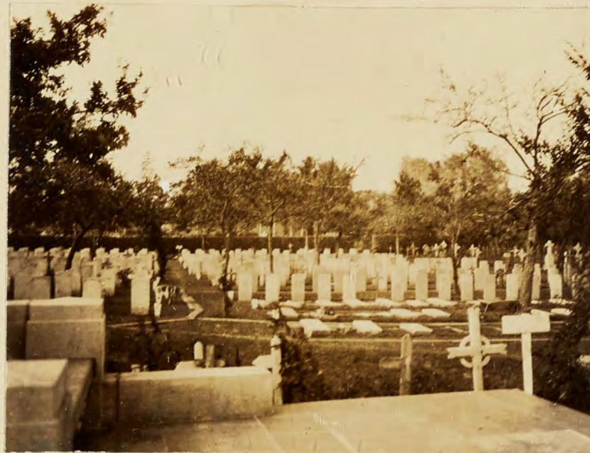
GENERAL VIEW FROM ENTRANCE.
