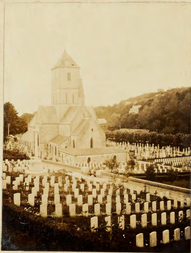
VIEW FROM RAILWAY EMBANKMENT
